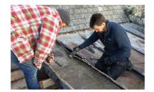
Removing the existing lead sheet proved difficult as it was very thick. It had to be cut into manageable pieces so that it could be removed.
