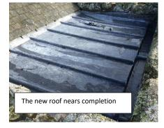
The new lead sheet is being laid in sections. Each section has to be shaped carefully despite its thickness
